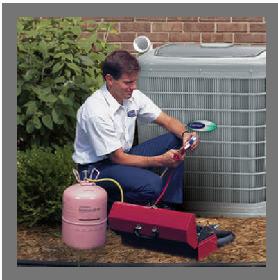
Air Conditioner Installation Service
